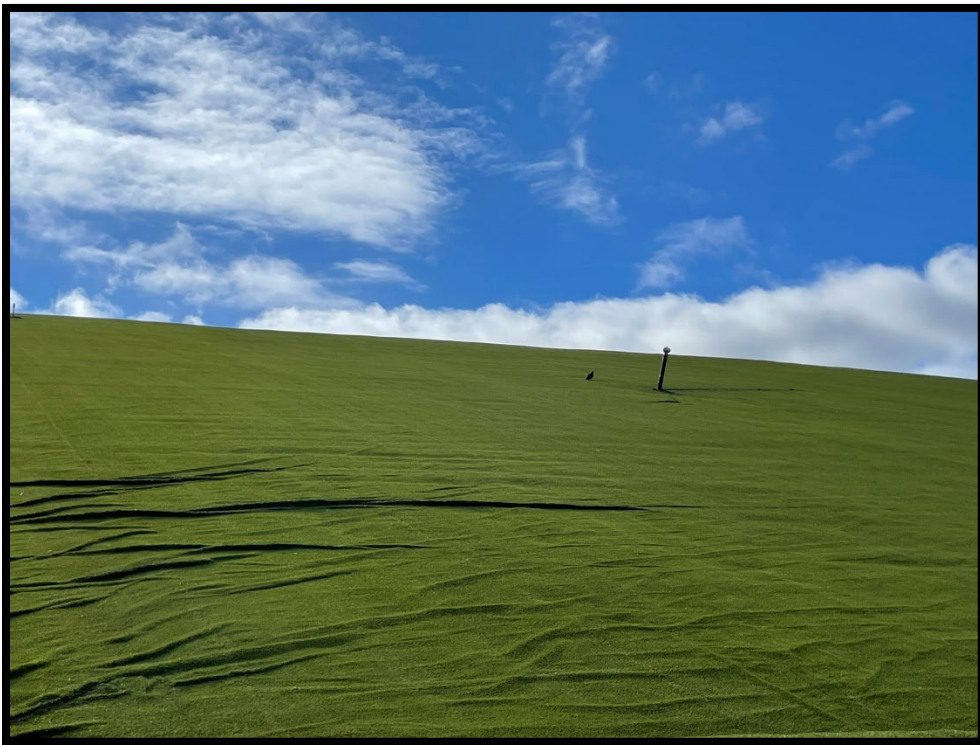
Photograph 4: View of damaged closure turf on the north side of Area 1-2.
