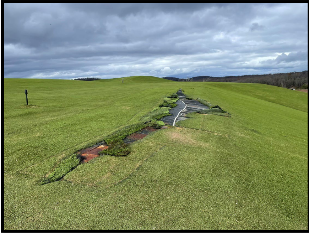
Photograph 5: View of damaged closure turf on east side of Area 1-3.
